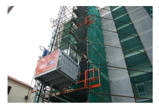
The TPL 500 has a payload capacity of 500kg and the TPL 300 can cope with loads up to 300kg. Both models have been designed to be flexible with interchangeable parts and the double tie frame arrangement makes them quick and easy to erect and dismantle. Although it is extremely robust in build, the 300kg machine is single phase and only
