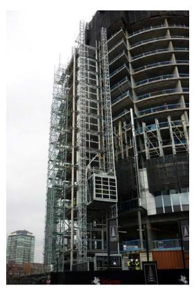
tested by RIFI, the CAS common tower has a mere 5 x 5 metre footprint yet is capable of running multiple hoists simultaneously. This allows all material and personnel hoists to be concentrated in one area, which streamlines loading efficiency at ground level. With all hoists operating simultaneously it minimises waiting times for men and materials, especially at peak times.
