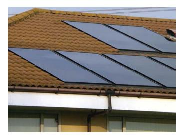
roofline remains flush and watertight. As well as being more aesthetically pleasing it means there is no additional load on the roof, so they can be fitted without any modification to the roof structure.
