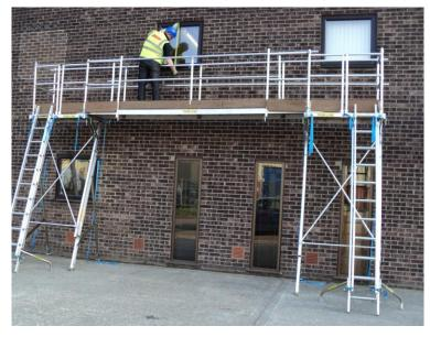
scaffolding is both slow to erect and too costly to justify for short duration jobs. Scaffold towers are too problematic in garden situations and uneven or sloping ground. Trim-Line has been designed to overcome all these issues. It is easy to transport, quick to erect and can cope with many of the access problems faced when fitting FSG including spanning conservatories, porches and bay windows.
